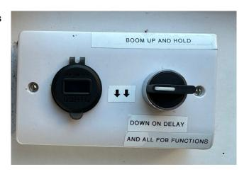
upright, open position and re-set the wait time delay before trying to close once again. The barrier will not respond to the fob while being held open by this control.
